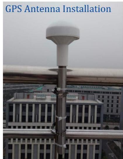
The server consists of the outdoor part and interior part. The outdoor part is composed of the GPS satellite receiving antenna, lightning arrester and antenna amplifier (optional). The function is to complete the reception of satellite signals.
